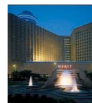
Hyatt Regency Indianapolis One South Capitol Avenue Indianapolis, IN
